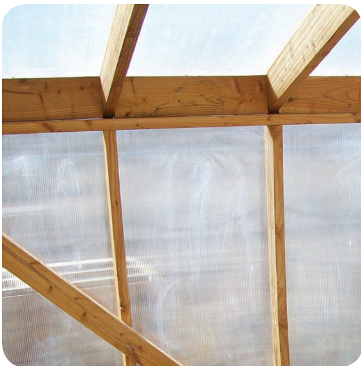
Greenhouse with Wooden Structural Support
